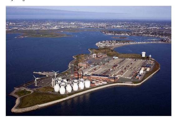
The plant was overhauled in the 1980's and 1990's at the cost of \$3.8 billion. Protecting the investment of that much money meant forward-thinking planning. Planners and engineers looked at the costs of elevating the plant by 1.9 feet, and compared it to the risks to the plant of future sea level rise. It would save money in the long run, they rationed, to elevate the plant now and prevent expensive fixes in the future – including elevating the sewage piping over a fortification wall.
